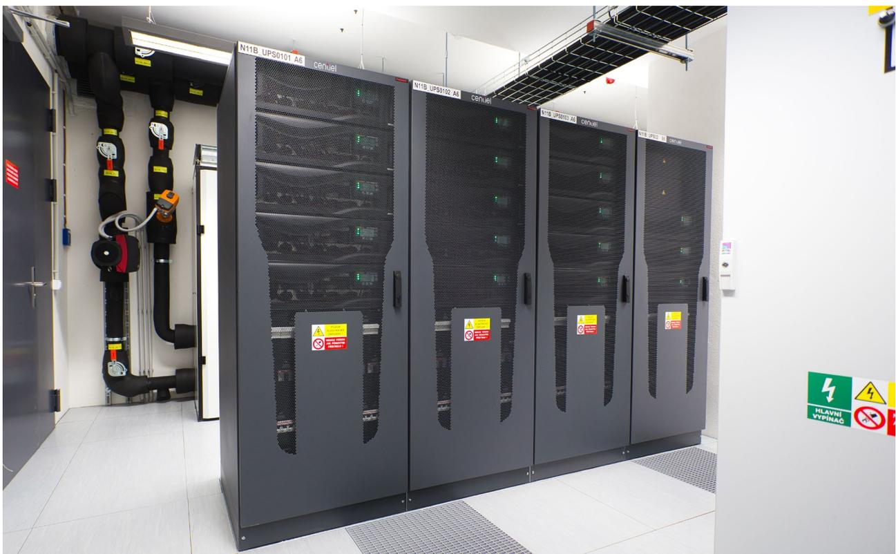
TTC TELEPORT's electrical power substation: Module 2, now sees the installation of 6 x CumulusPower™ 300kW frames populated with 12 x 60kW Intelligent UPS Modules (IM) and 1 x CumulusPower™ 300kW frame populated with 3 x 50kW IM. These units will support the IT and control and monitoring elements of the datacentre.
