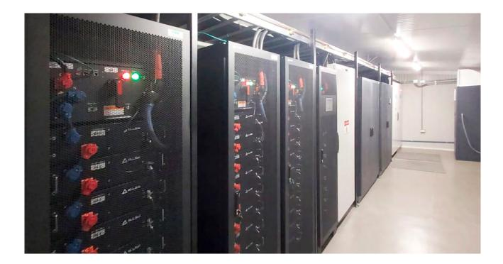
straightforward to set up. Servicing is easy as each individual module can be evaluated or hot-safe-swapped without compromising the load or the system.
