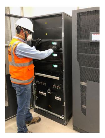
The two 180kW CumulusPower<sup>™</sup> units were set up in parallel (2x3xIM60) with battery banks made up of four cabinets each containing 200 batteries, to provide a 30-minute run time at 75% load. The installation took four staff just 15 days to complete.
