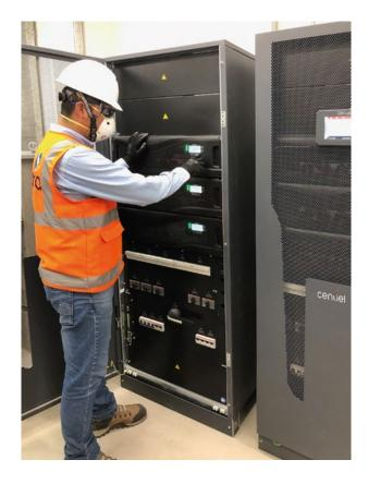
The two 180kW CumulusPower™ units were set up in parallel (2x3xlM60) with battery banks made up of four cabinets each containing 200 batteries, to provide a 30-minute run time at 75% load. The installation took four staff just 15 days to complete.
